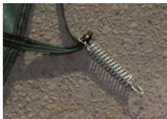
Fixing by spring + stainless steel piton
