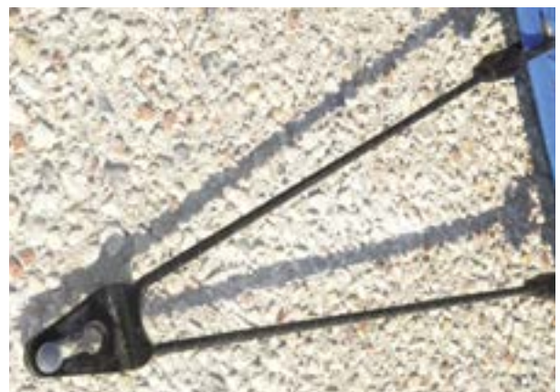
Fixing by Sandow SPPE 60 cm + Piton socket
